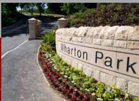
▼ ESH – WHARTON PARK, DURHAM. HERITAGE CENTRE, CAFÉ FIT-OUT & STONEMASONRY
