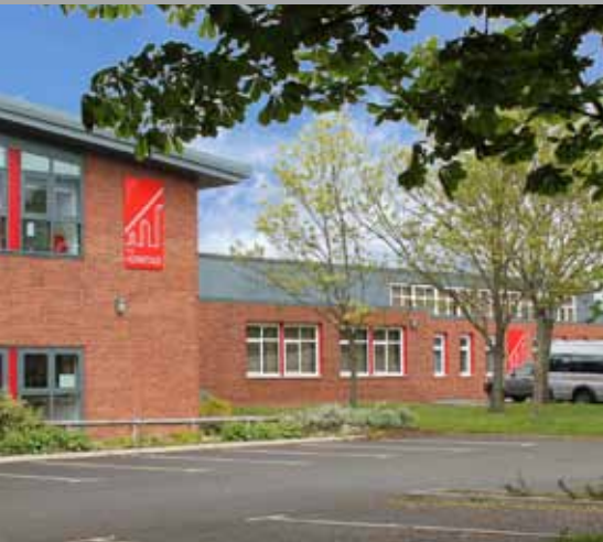
▲ HERMITAGE ACADEMY, CHESTER-LE-STREET. NEW 6TH FORM BLOCK
